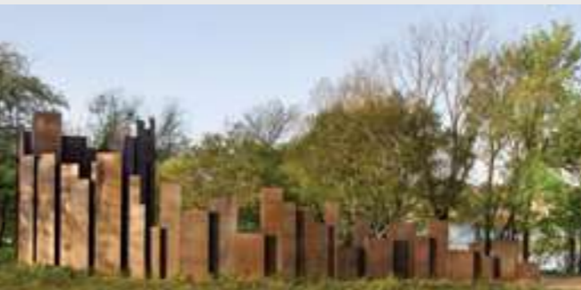
Trail Restroom - Arch. Mirò Rivera
