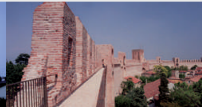
RENOVATION PRIZE: City walls of Cittadella - Patrizia Valle
