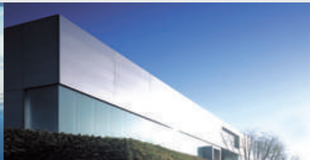
Metal Office - Tokashi Yamaguchi & Associated
